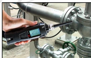
For gas pipe joint
